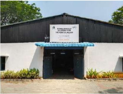
Training Academy main building
