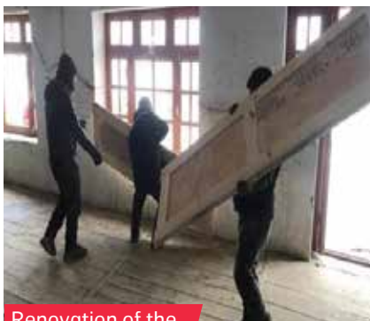
Renovation of the community centre
